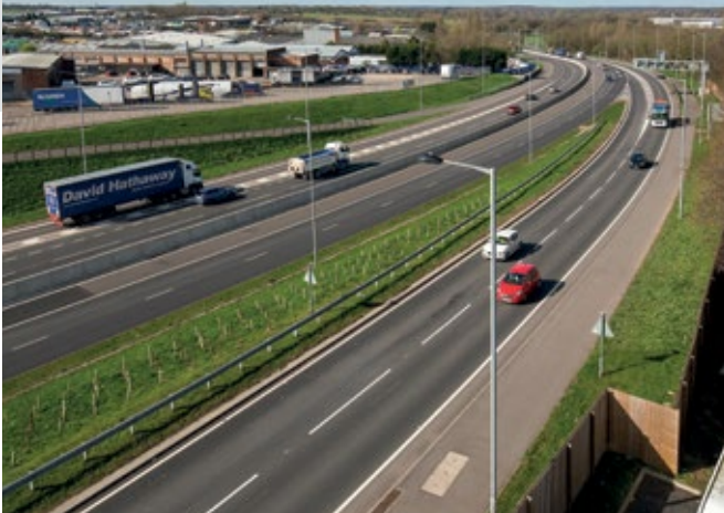
Our £106m improvement scheme built at Tollbar End in Coventry
